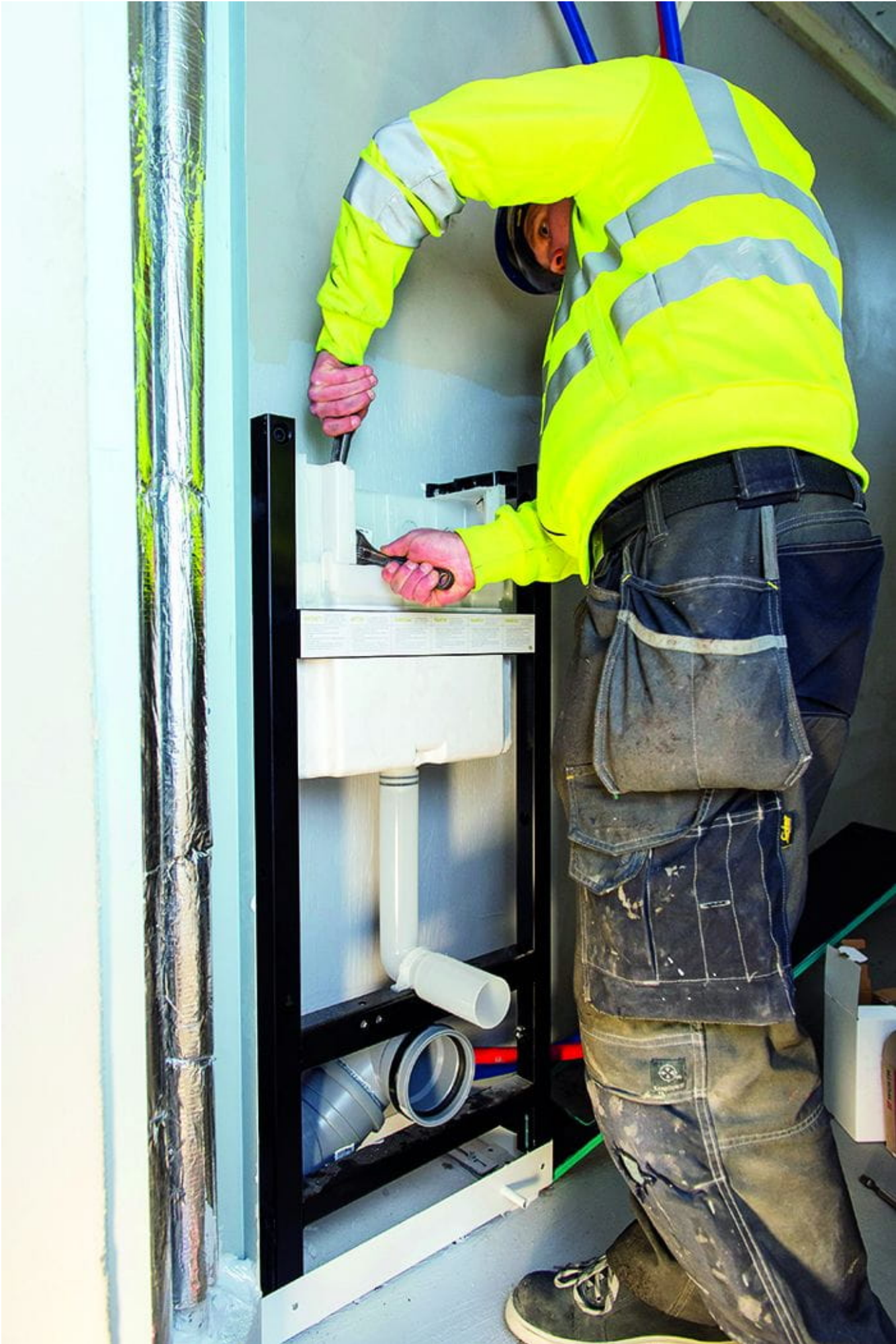
A housing company in Turku saved time and money using Uponor's Cefo pipe overhaul
