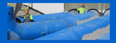
Underground ventilation pipes and fittings dimension 1200 mm
