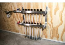
Besides offering a higher flow velocity compared to CPVC or copper, a PEX system holds a smaller volume of water than the same-sized system using either of these materials in the same pipe diameters.
