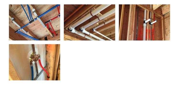
PEX is more forgiving and it's lighter than copper. We used to use CPVC, stainless and copper pipes, but ProPEX fittings, man, it's quick and fast.
