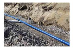
The pipes are light and flexible, thanks to which they are easy and fast to install. Their flexibility also means that small changes in direction can be implemented safely.
