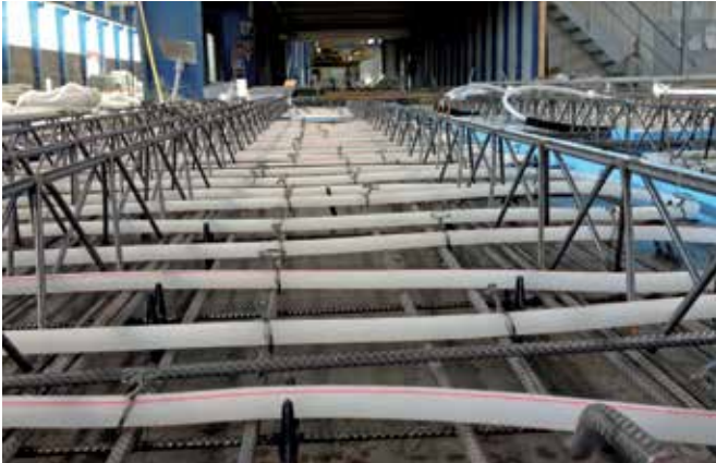
Pipes positioned in the prefabricated filigree slab before the concrete pouring.
