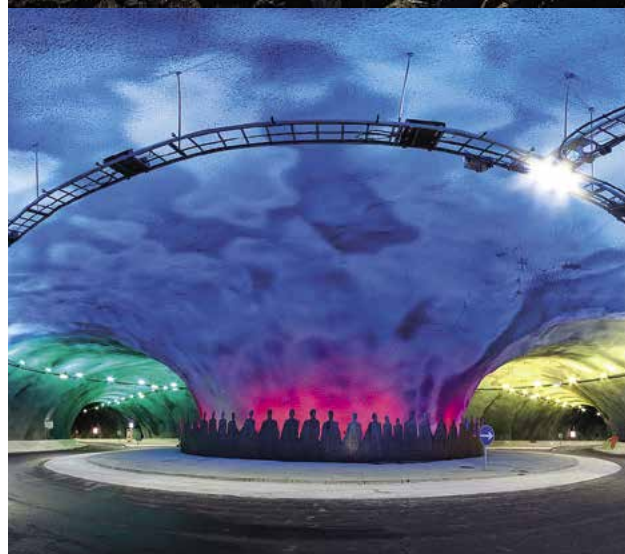
The 11.2-kilometre tunnel runs at its deepest 189 metres below sea level.
