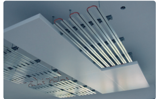
Heating/cooling coil with magnet technology suspended on threaded rods. Subsequent mounting of ceiling panels complete the ceiling island.
