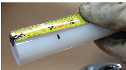
Figure 3-27 Measure from End of Pipe
