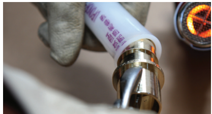
Figure 3-25: Work Piping Back and Forth
