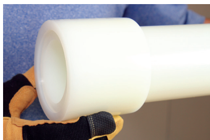
Figure 3-15: Ensure Ring Reaches Stop Edge
