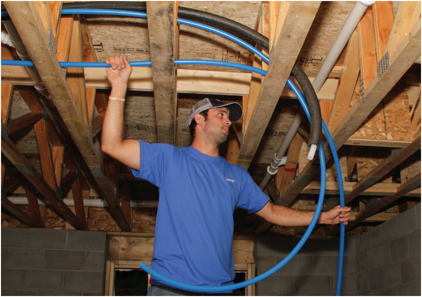
Figure 6-1: Running Uponor AquaPEX Main Lines Through Open-Web Trusses
