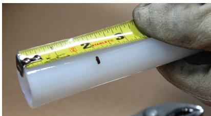
Figure 3-27 Measure from End of Pipe
