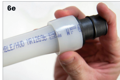
Figure 3-5: Inserting ProPEX Fitting into 1" Uponor PEX Piping
