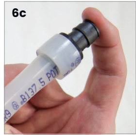
Figure 3-4: Inserting ProPEX Fitting into 1/2" Uponor PEX Piping
