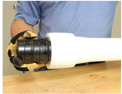
Figure 3-18: Insert Fitting
