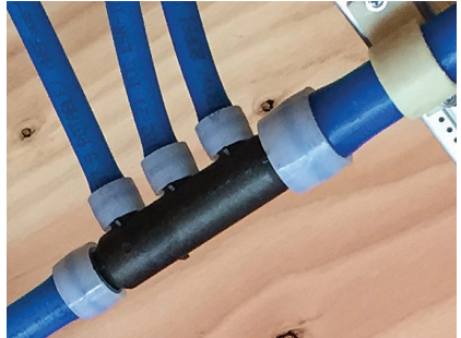
Figure 6-9: Multiport Tee Installation
