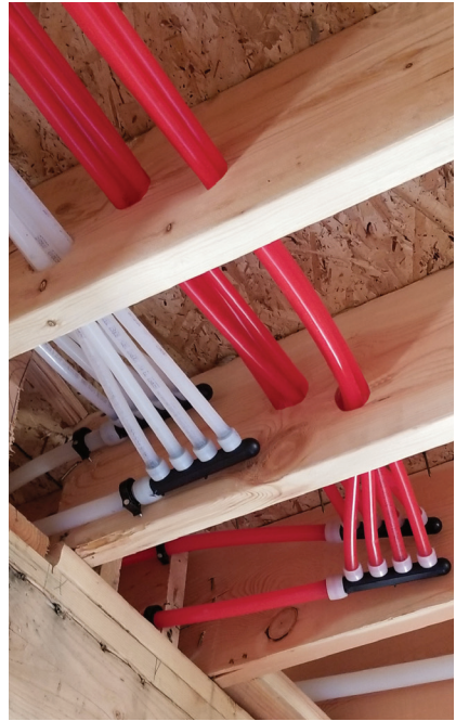
Figure 6-7: Bundled Uponor AquaPEX Pipe
