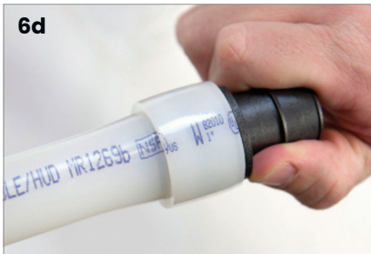
Figure 3-5: Inserting ProPEX Fitting into 1" Uponor PEX Piping
