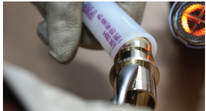
Figure 3-25: Work Piping Back and Forth
