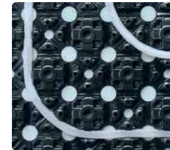
Uponor PE-Xa pipe installed at 90° angle
