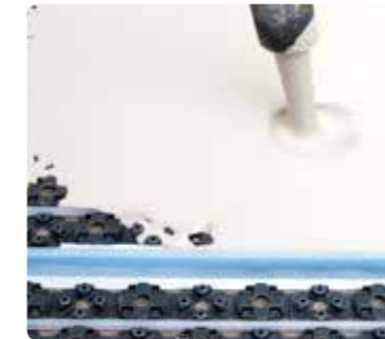
Levelling compound can spread easily
