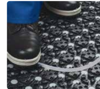
Cost-saving one-man installation
