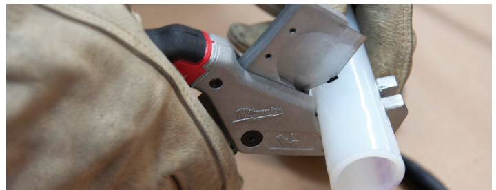
Figure 2-39: Cut pipe at marking
