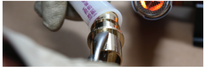
Figure 2-36: Work piping back and forth
