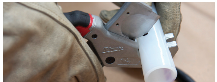
Figure 2-39: Cut pipe at marking
