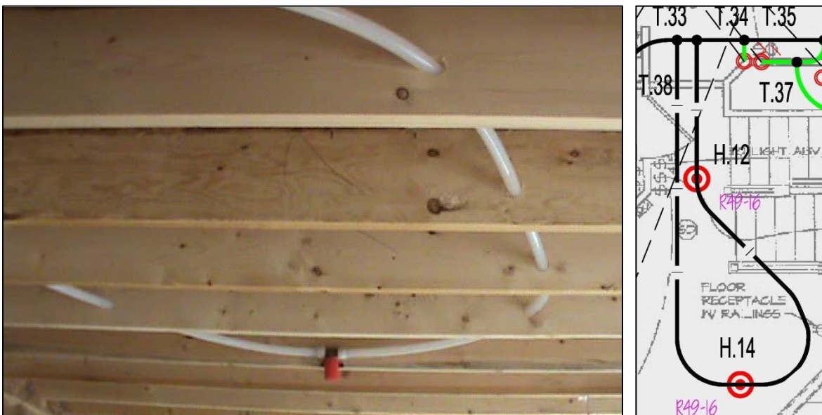
Figure 3: Sub-loop Air Pocket
