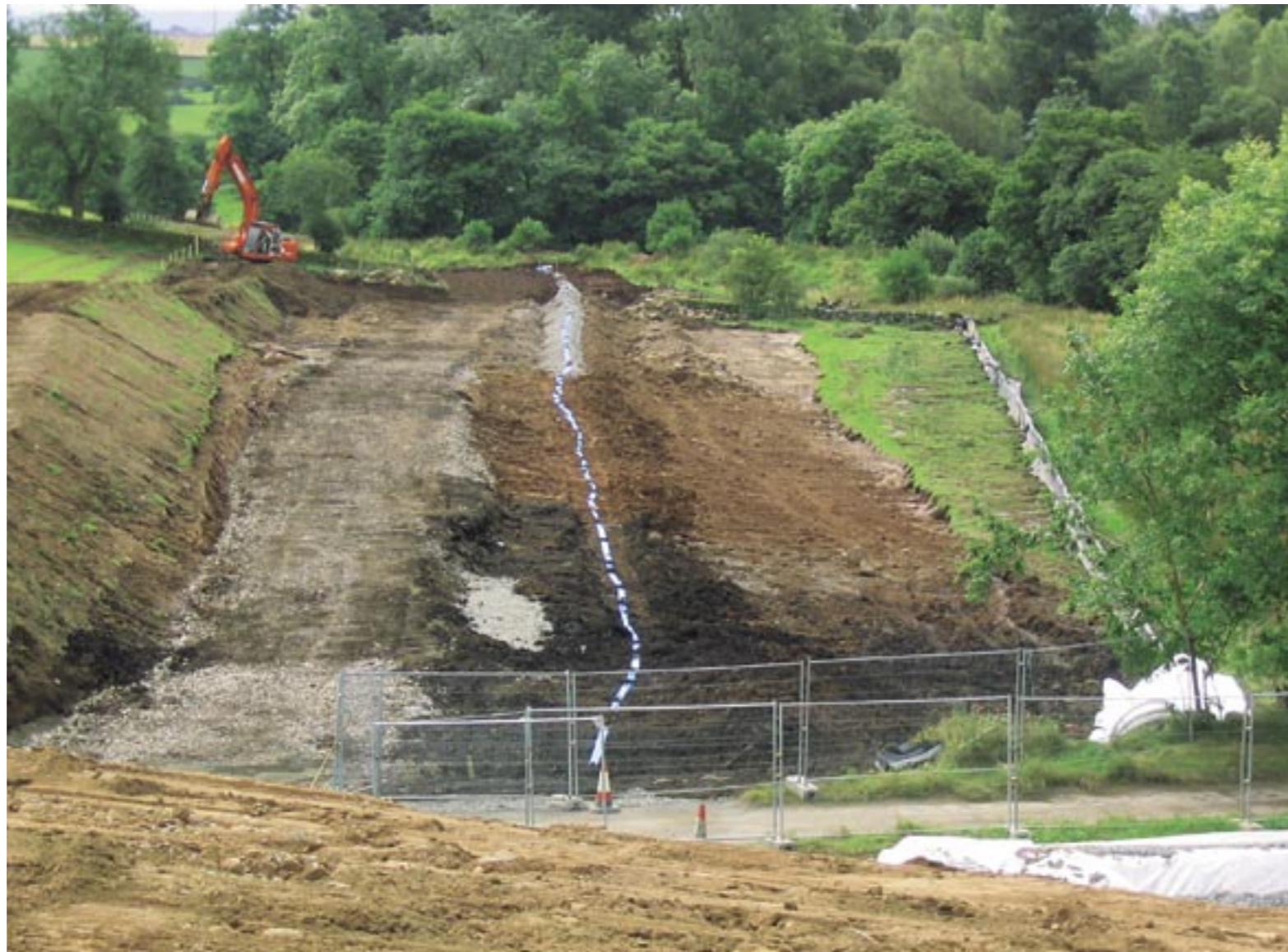
The new £120 million water treatment works at Mugdock will ensure the clean water supply for the City of Glasgow for years.
