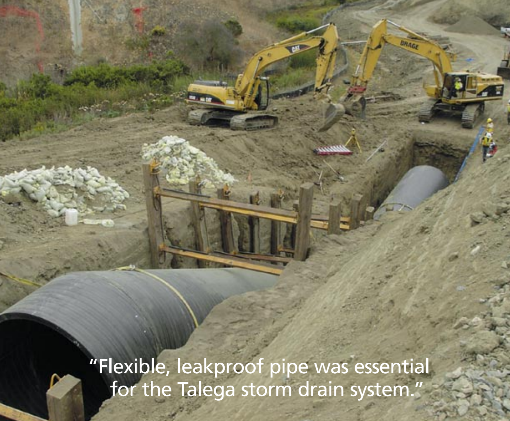
Talega, California, storm drain slithers like a snake down the valley incline for 6,700 feet.
