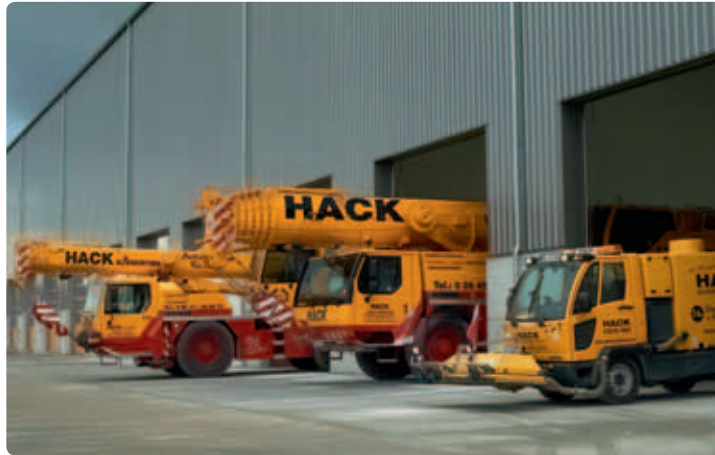
Hack Heavy Duty Vehicles Maintenance Facility, Windhagen, Germany. Equipped with Uponor industrial underfloor heating.
