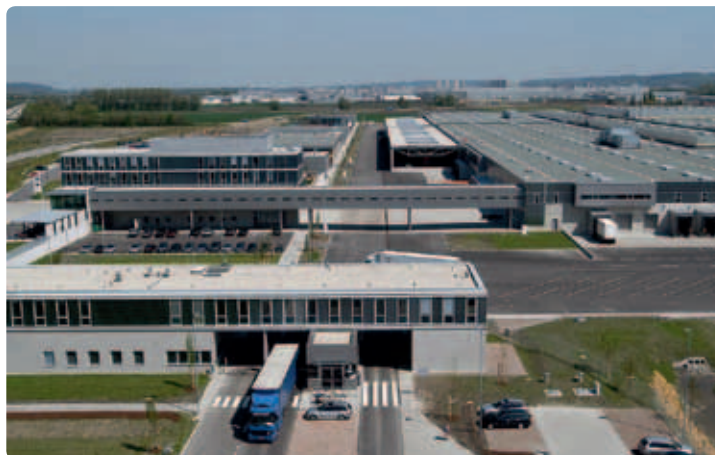
BMW Dynamic Center, Dingolfing, Germany. Equipped with Uponor industrial underfloor heating.
