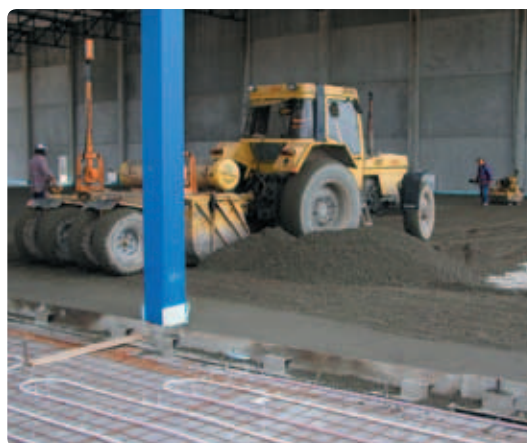
Using roller compacted concrete.
