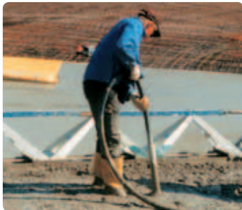
Concrete compaction using vibrating cylinders
