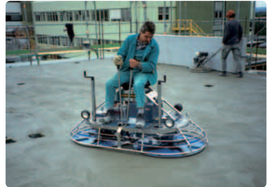
Rotor-type power trowel for smoothing of concrete surfaces
