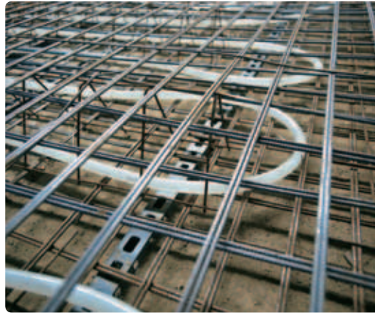
Reinforced concrete with mesh reinforcement.
