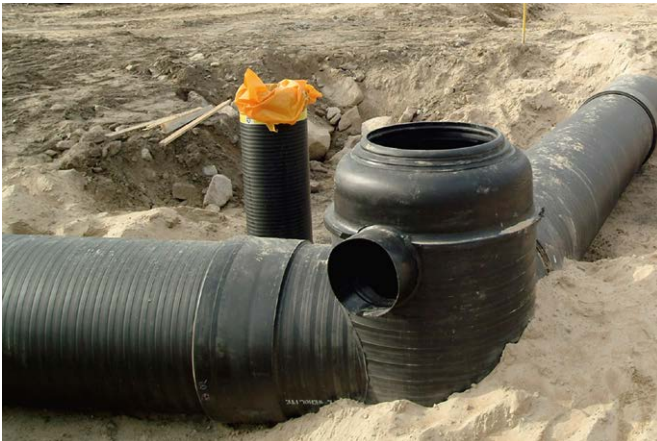
Ilmajoki, Finland: The total length for the waste deposit collector pipeline is more than 2550m and it consists of Weholite pipes DN/ID 600 and 700mm, stiffness class SN4.
