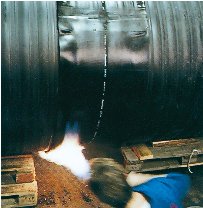
Heat shrink sleeve installation
