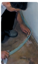
Uponor Minitec Installing edge strips
