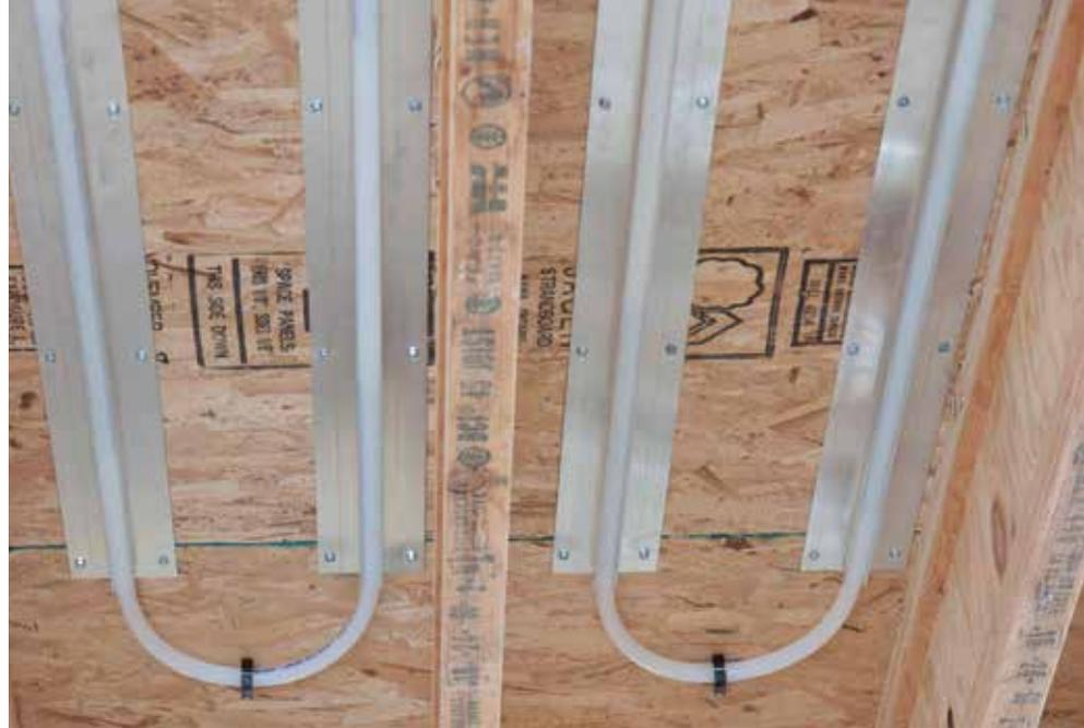
Figure 7-4: Joist Trak aluminum heat transfer plates
