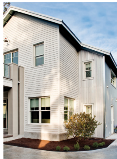
Green builder VISION house 2011, Orlando Florida, USA: Uponor's plumbing and sprinkler systems were used at the VISION house, which explores green building and sustainable living options.
