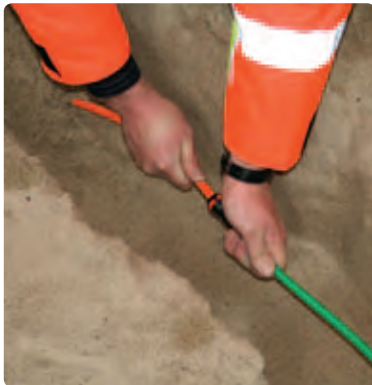
7. Fit a single Opto Net duct into the connector and pull it through.
