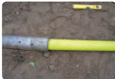
Figure 8.2.24. Slotting the Tripla pipe into the mole head.
