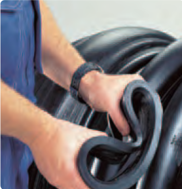
2. Install the PE inlet in the hole.
