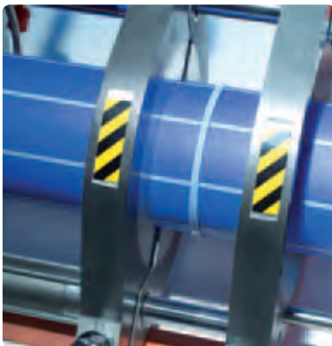
A successful joint showing a visible, high bead.
