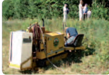
Figure 8.2.28. A 12 m road crossing carried out by horizontal drilling
