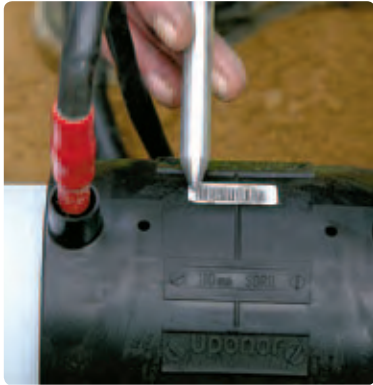
7. Enter the welding data using the barcode system.
