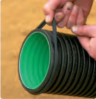
2. Fit the sealing ring onto the first groove from the spigot end.
