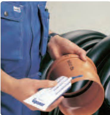
3. Apply lubricant to the socket pipe.
