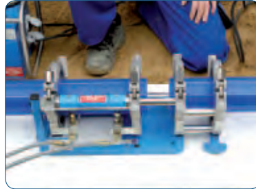
Figure 8.2.33. Butt-welding ProFuse pipes.
