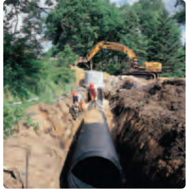
6. Initial backfill must be evenly compacted on both sides of the pipe. Uneven compaction can result in the transverse displacement and deformation of the pipe.
