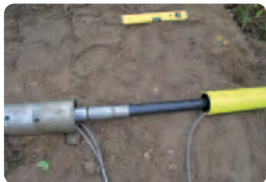
Figure 8.2.23. Fastening the Tripla pipe to the mole.
