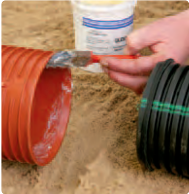
3. Apply lubricant to the inside of the socket.
