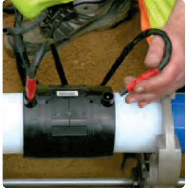
6. Set up the welding cables. The socket is now ready for welding.
