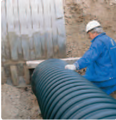
5. The pipes are coupled by pushing the spigot end fully home to the base of the socket. If an excavator bucket is used to push the pipe into place, always place a block of wood between the bucket and the pipe. The pipe must not be cut.
