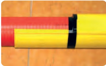
Figures 8.2.17 and 18. Repairing a damaged Tripla pipe using the split pipe method.
