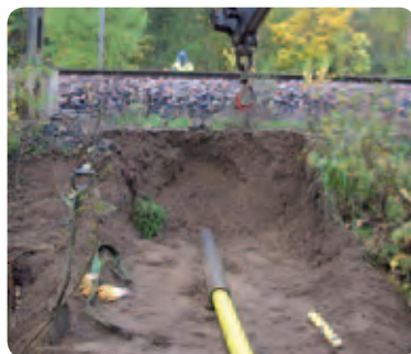
Figure 8.2.26. A completed pipe crossing.
