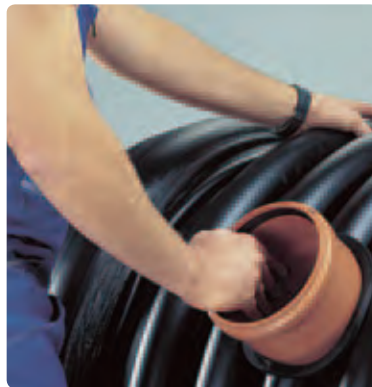
4. Install the socket pipe.
