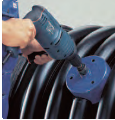
1. Drill the inlet hole with a hole drill.
