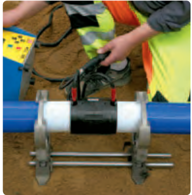
8. Carry out the electrofusion.
