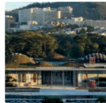
Planted roof on top – Uponor heating and cooling system inside
