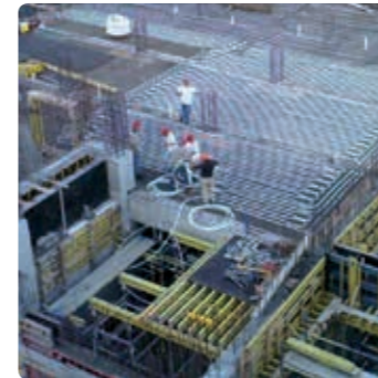
Laying of the pipe mats
