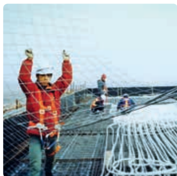
Installation of the TABS modules
