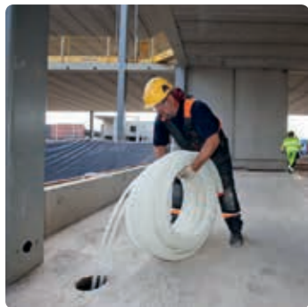
Uponor PE-Xa pipes are integrated into the energy piles, which are then concreted. Ground-source energy then transfers to the heat exchange fluid in the piping. Energy piles both heat and cool the building
