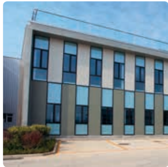
The zero emission building houses the administration of the Bayer MaterialScience plant
