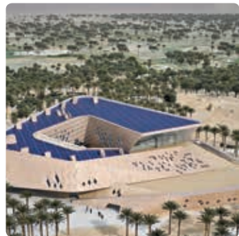
High cooling loads of 1.5 MW are mainly delivered from the Uponor TABS of 7,500 m²
