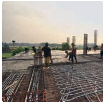
Installation of Uponor TABS radiant cooling
