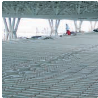
Its 150,000 m 2 of cooled floor area is recognised as the world's largest application. With the length of 440 m and a width of 110 m and an area of almost 500 000 m 2 the terminal became the largest combined building complex of its kind in the world
