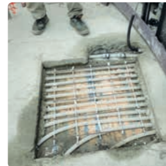
Approval of the underfloor cooling installation in June 2011
