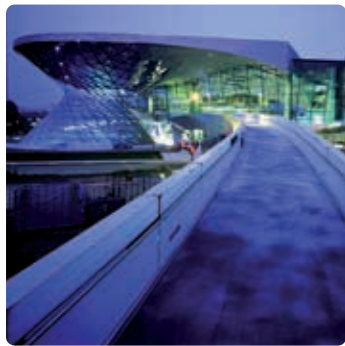
The construction incorporates a range of smart Uponor systems
