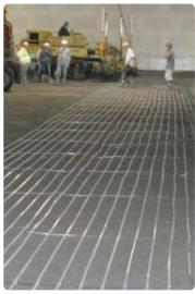
With the Radiant Rollout Mat, six contractors installed 35,000 square feet (16 to 19) mats per day. Installing the Uponor Radiant Rollout Mat covered 7.7 times more square footage when compared to conventional installation methods for a store this size.
