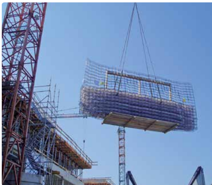
Proper crane transport of a Contec module pack with upright modules
