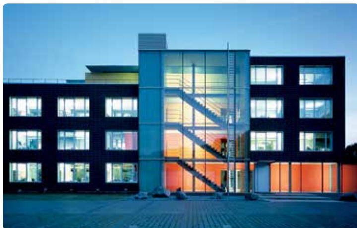
BOB - Balanced Office Building, Aachen, Germany, 2.000 m 2 Uponor Contec
