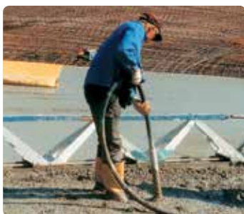
Concrete compaction using vibrating cylinders
