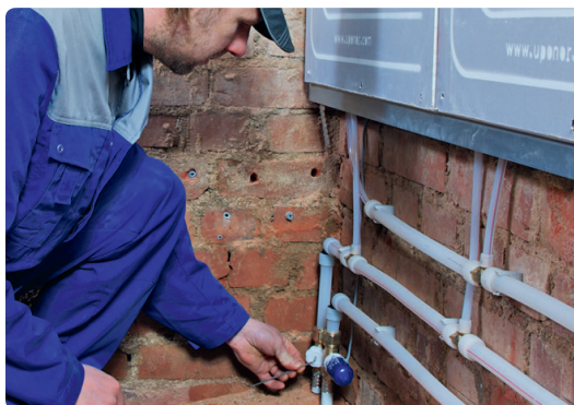
Example: Connection of Uponor Renovis panels mounted on the wall. Single room control by room thermostat.
