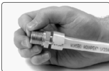
Figure 4-8: Remove the Expander Tool
