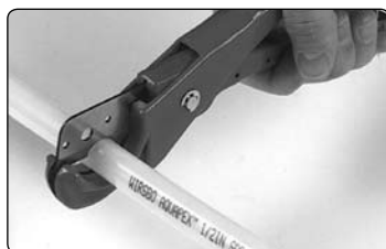
Figure 4-1: Square-cut the PEX Tubing
