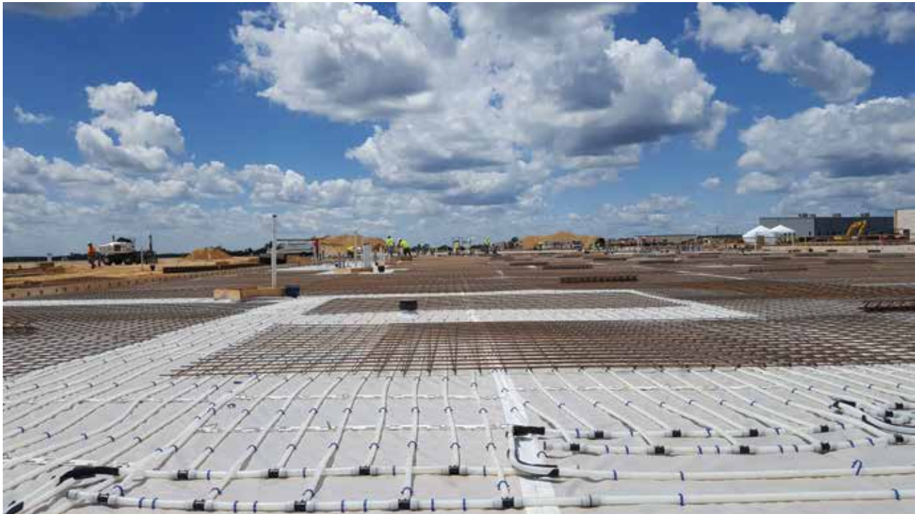
Figure 10-8: Radiant Rollout Mat featuring reverse-return header with piping module
