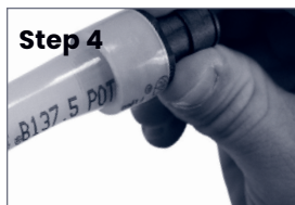
Figure 6: Insert fitting
