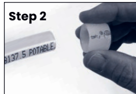
Figure 4: Slide ProPEX ring onto pipe
