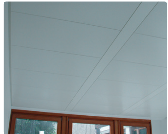
Sheet metal heating/cooling ceiling with VARICOOL Spectra as a bandrastrer construction
