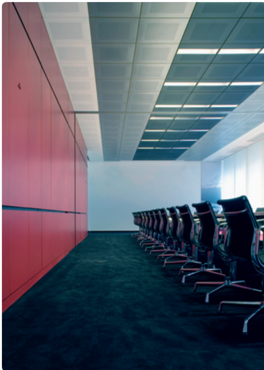
Cassette heating/cooling ceiling with standard spacing 625 mm special perforation and recessed lighting
