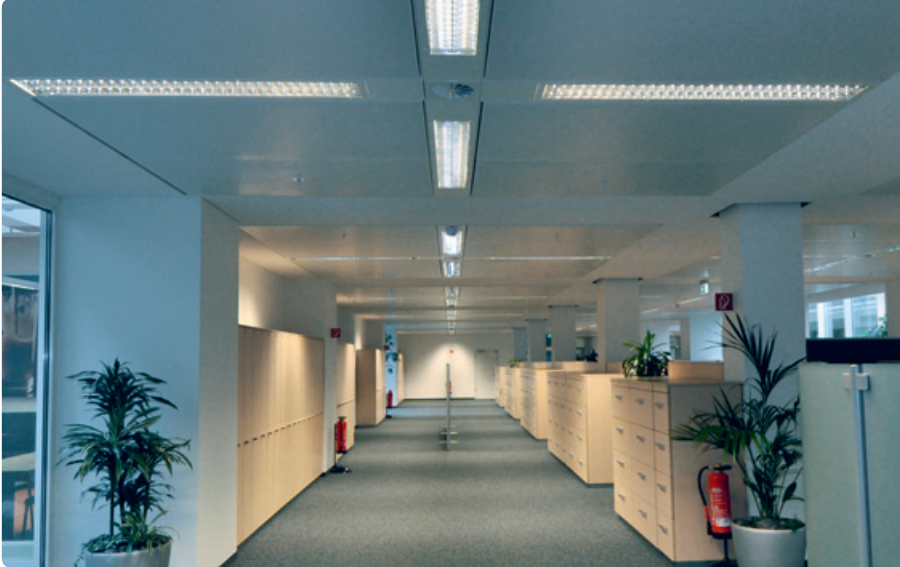
VARICOOL Spectra heating/cooling ceiling system as a closed metal ceiling
