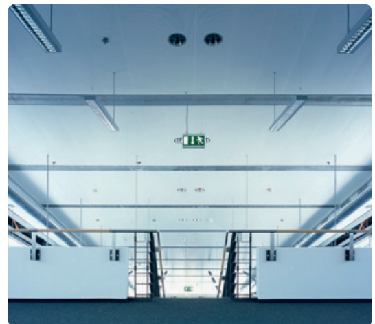
Sheet metal heating/cooling ceiling with VARICOOL Spectra in combination with various fixtures such as sprinklers, smoke detectors and pendant lighting
