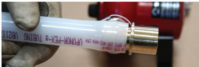
Figure 2-35 : Chauffer le raccordement
