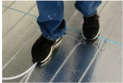
Figure 13: Press pipe into the groove
