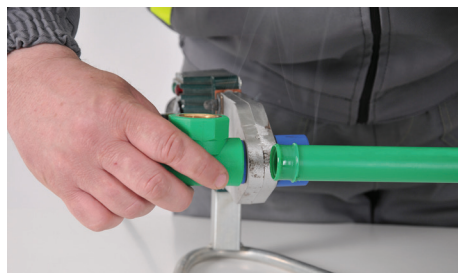
Figure 2-4: Connecting the pipe and fitting
