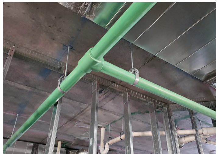
Figure 1-4: PP-RCT suspended piping
