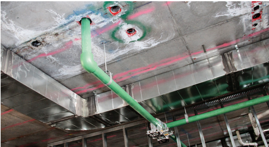
Figure 3-1: Ceiling penetration
