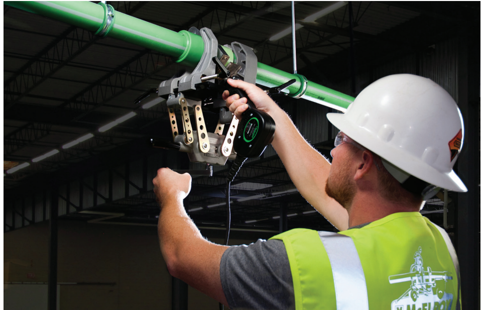
Figure 5-1: Making overhead PP-RCT connections
