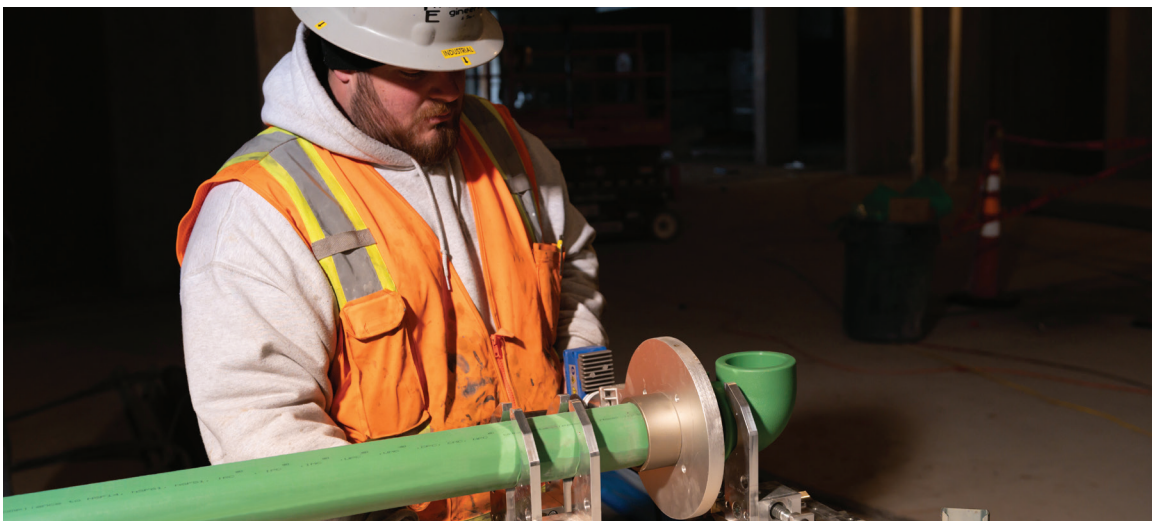
Figure 2-1: Heat-fusion connection
