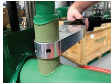
Figure 2-8: Heating a saddle outlet
