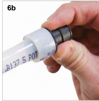
Insert ProPEX fitting into 1/2" Uponor PEX piping.
