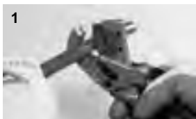
Figure 5: Square cut the pipe.
