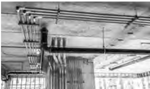
Figure 31: Supporting PEX with PEX-a Pipe Support
