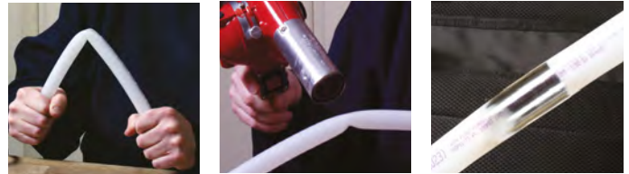
Figure 6-3: Reforming kinked piping
