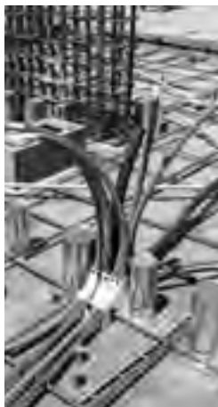
Figure 55: In-slab installation
