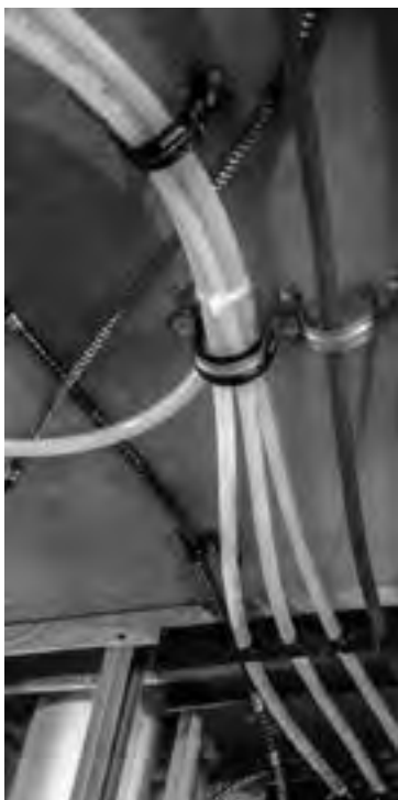
Figure 30: Proper bundling of Uponor PEX
