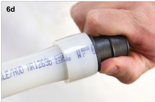
Insert ProPEX fitting into 1" Uponor PEX piping.
