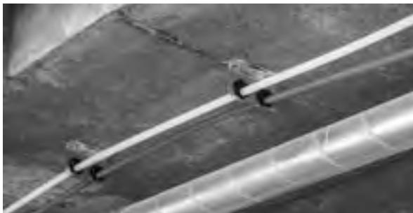
Figure 24: Supporting small-diameter coiled PEX
