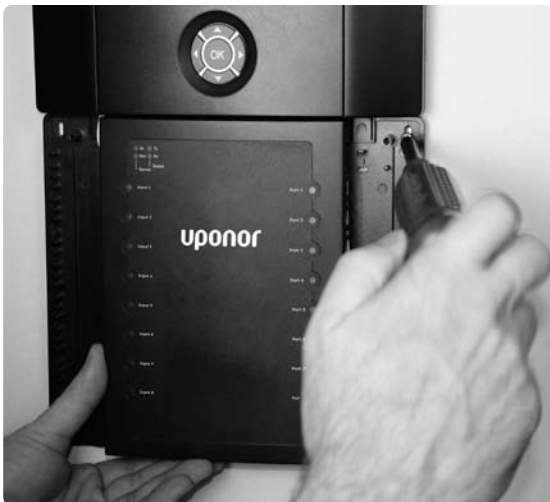
Figure 3-1: Installing Initial Screw
