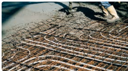
In situ concrete casting
