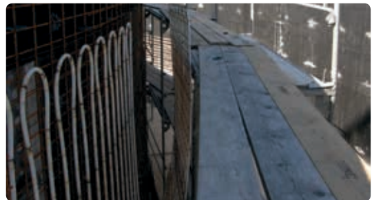
Uponor Contec modules installed in wall
