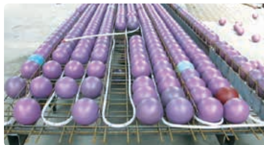
Cobiax® modules, coupled with Uponor Contec system as precast modules
