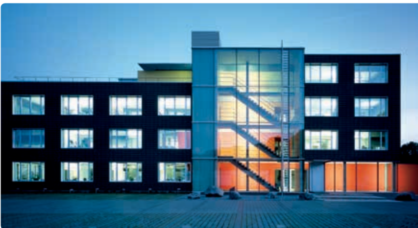
BOB-the Balanced Office Building, Aachen, Germany, 2,000 m 2 Uponor Contec
