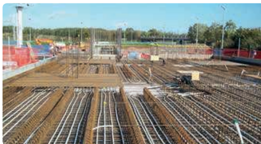
Floor section of U-Boot® with Uponor Contec system
