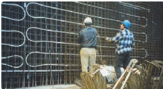
Uponor Contec modules installed in wall
