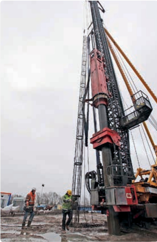
Installing the reinforcing cages
