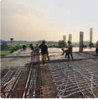
Installation of Uponor TABS radiant cooling
