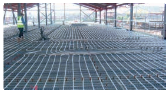
Uponor Contec installed in metal deck
