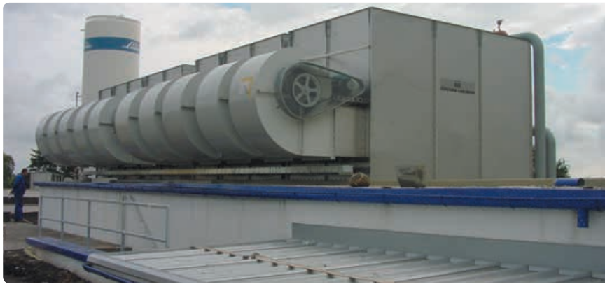
Utilisation of recooling units for generating cold water
