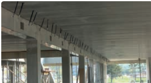
Uponor Contec modules incorporated into precast hollow core
