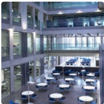
A low energy University building incorporating thermal mass, natural daylight, controlled ventilation, a number of integrated energy generation features and ground source heat pumps
