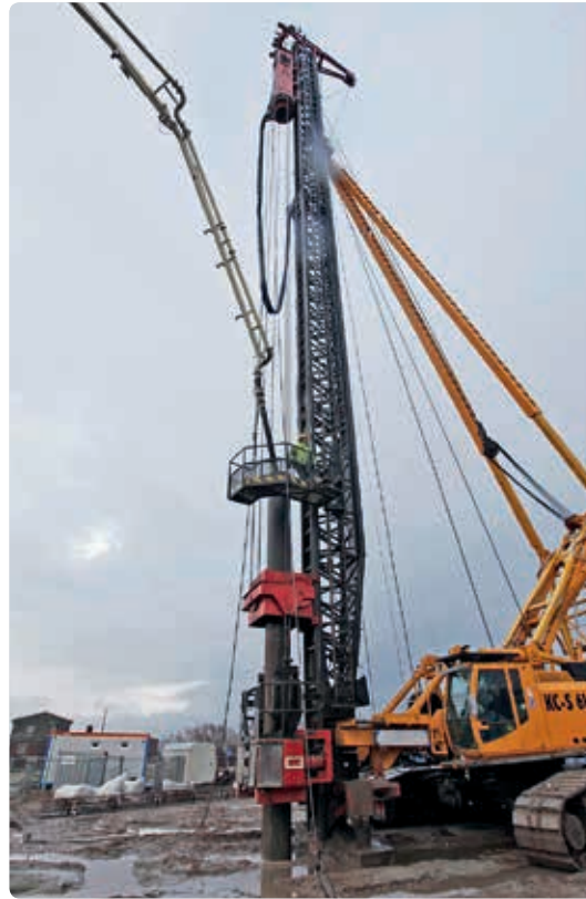
Concreting procedure of the in-situ piles
