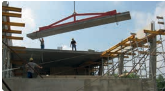
Crane transporting the precast concrete slab element to the correct position
