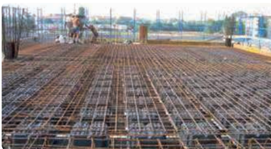
Uponor Contec installation, concreting and U-Boot modules installation
