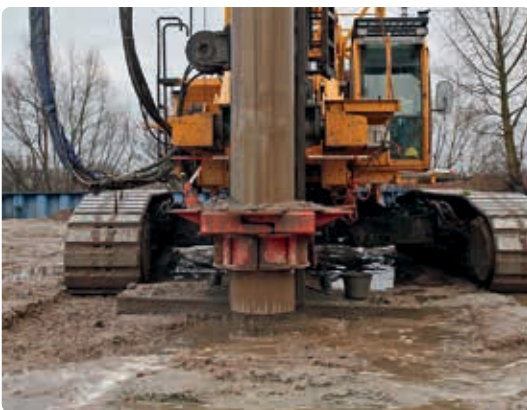
Assembly of a bore pile
