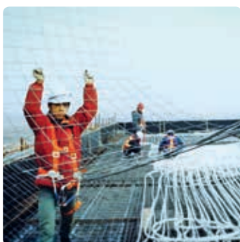
Installation of the TABS modules
