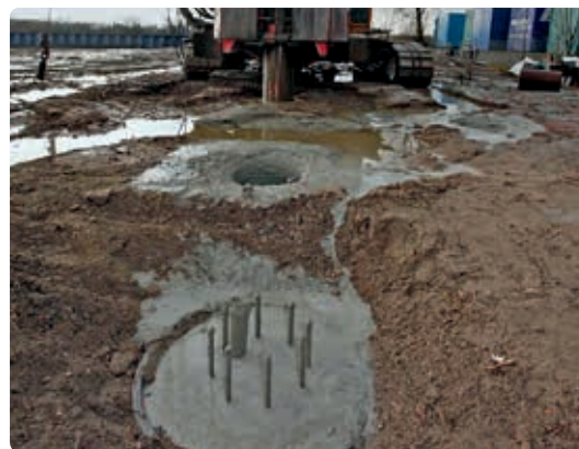
Prefabricated concrete bored pile
