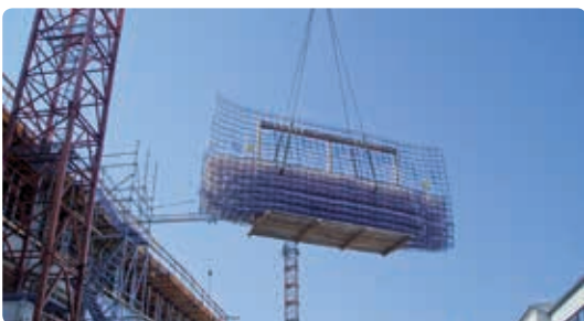
Proper crane transport of a Contec module pack with upright modules
