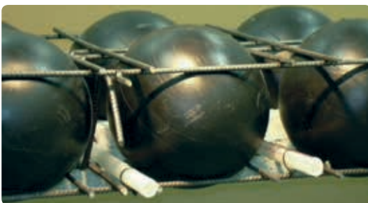
Floor section of Cobiax® modules with Uponor Contec
