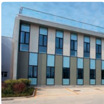
The zero emission building houses the administration of the Bayer MaterialScience plant
