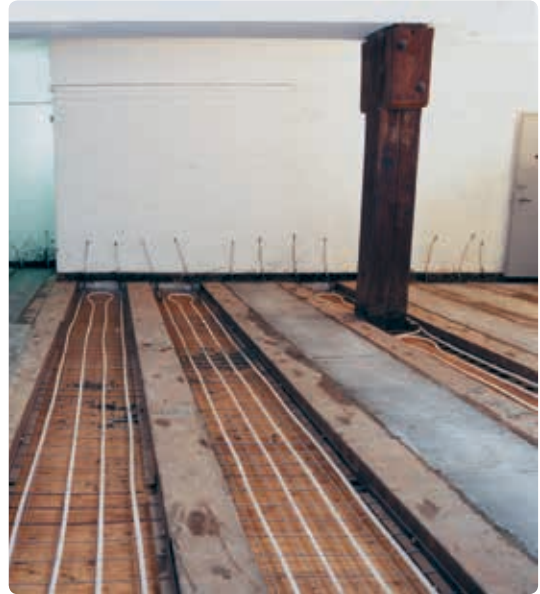
Tailor-made installation between ceiling beams
