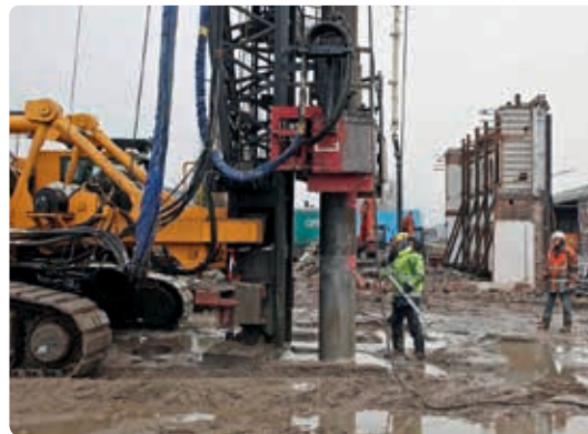
Supervision of the pile assembly
