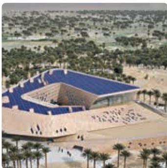
High cooling loads of 1.5 MW are mainly delivered from the Uponor TABS of 7,500 m 2
