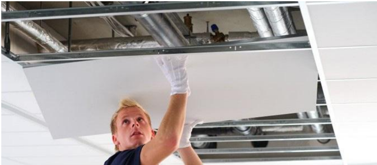
Uponor Comfort panel for ceiling cooling and heating
