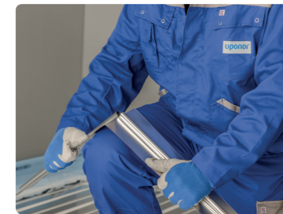
Divide the heat conduction plate by bending it only
